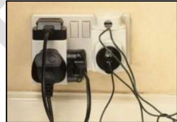
The use of extension cables, trailing leads and adaptors to power portable appliances should be avoided wherever possible.
